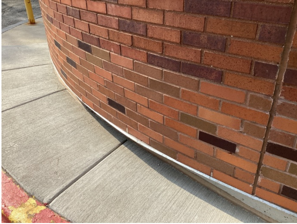
Base flashing installed
