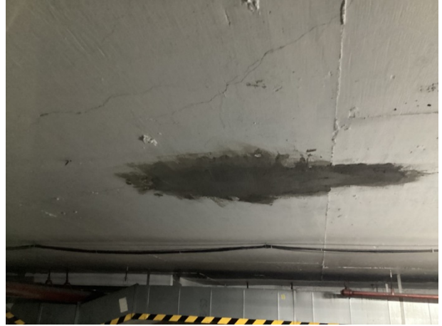
Concrete repairs beneath 1P
