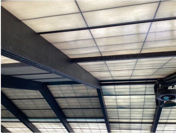
Pool enclosure roof
