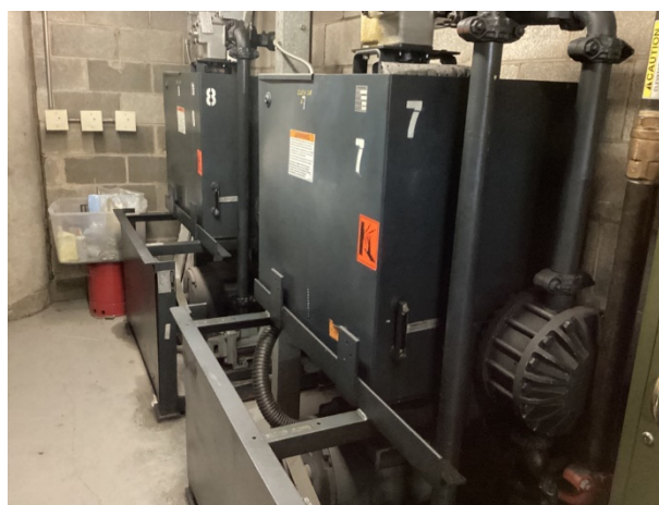
Mall/garage elevator casings
