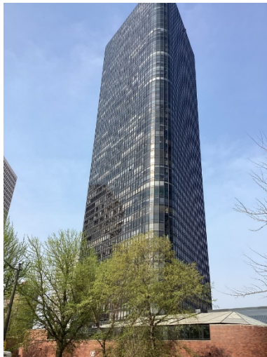
North and east elevations
