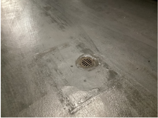
Traffic coating at drain
