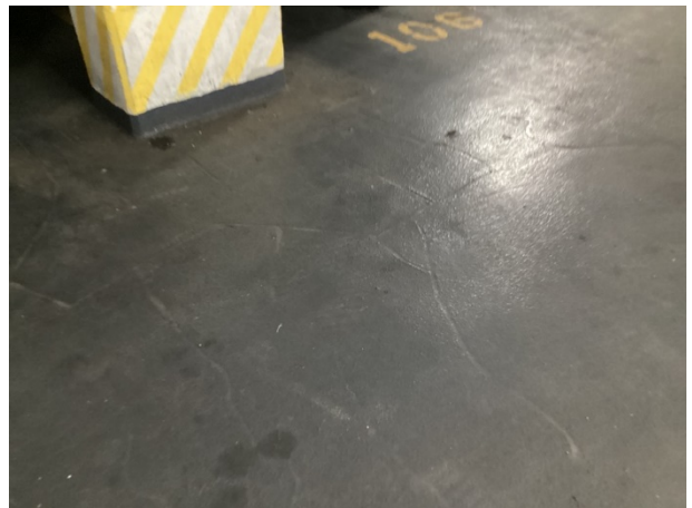
Concrete repairs beneath traffic coating
