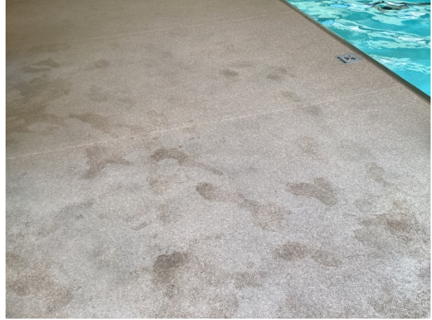
Pool area flooring
