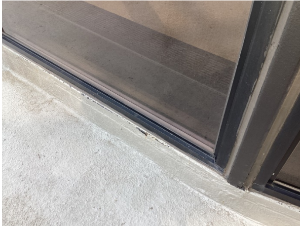
2 nd floor walkway window system
