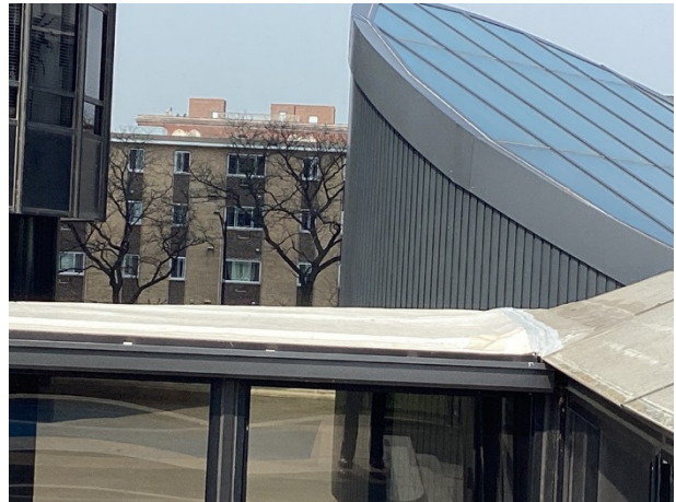
Walkway roof at 2nd floor
