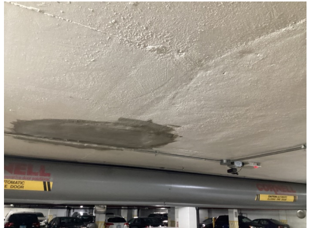
Concrete repairs beneath 1P
