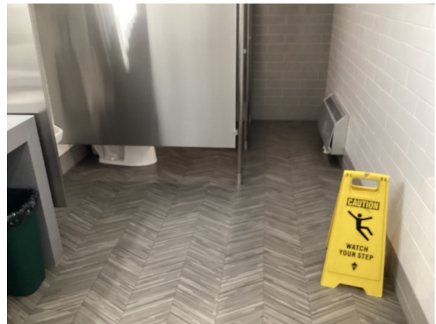
Rest room at mall
