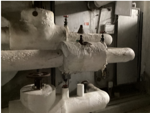
Lobby air handling unit
