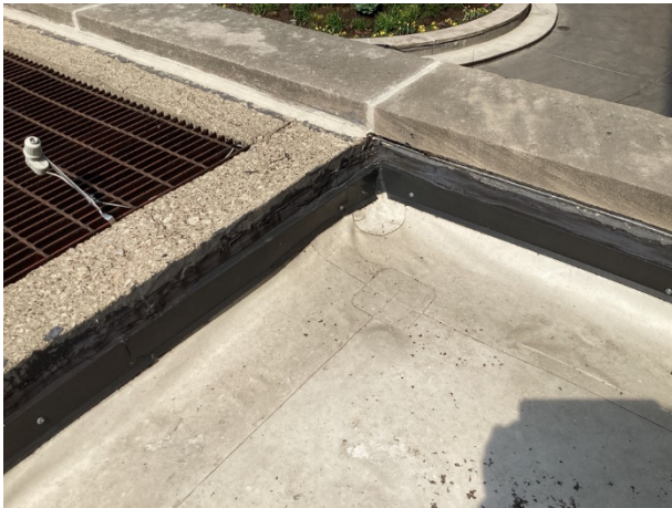
Southwest roof at 2nd floor at perimeter
