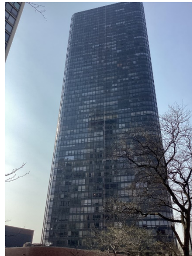
North and west elevations
