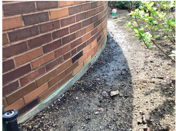
Flashing at planter at 2nd floor
