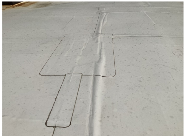
Northwest roof repairs at 2nd floor
