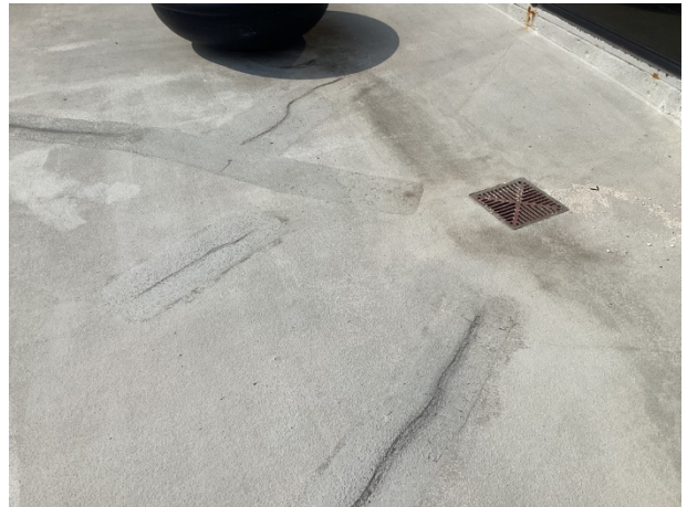
Repaired cracks at 2nd floor roof
