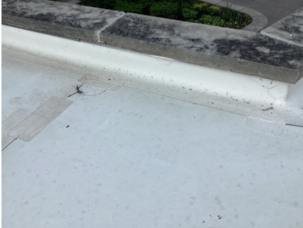
Perimeter at 2nd floor northwest roof
