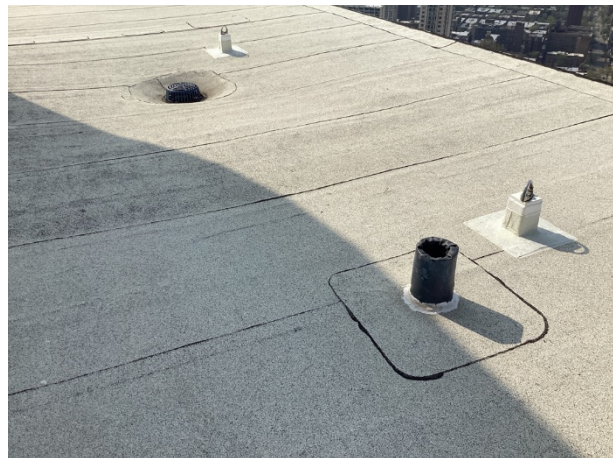
Main roof at penetrations
