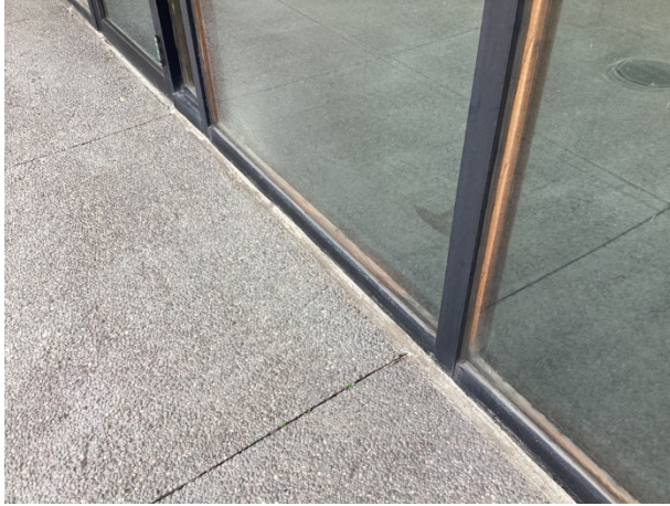
Mall window system (commercial owner responsibility)
