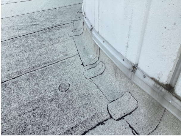
Main roof at perimeter repairs
