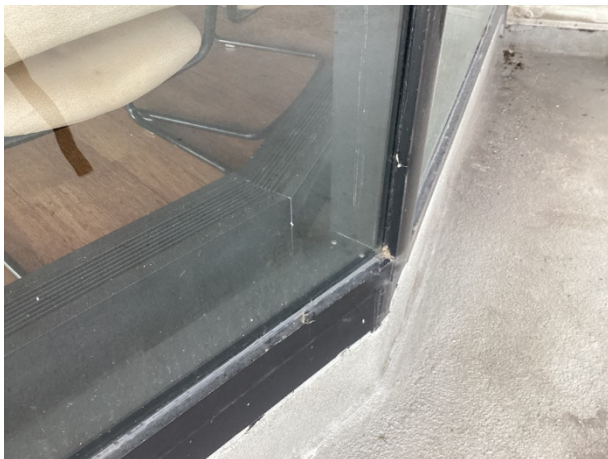
Party room window system
