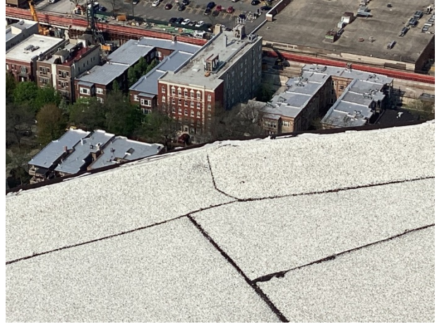
Main roof at perimeter sealant
