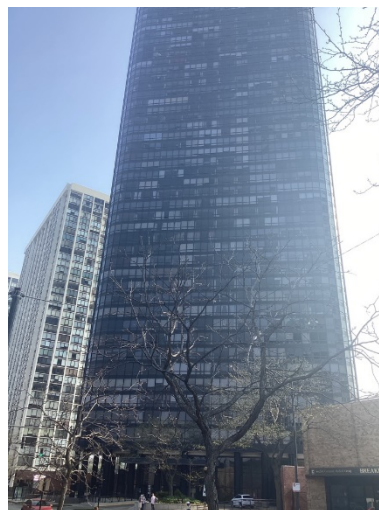
South and west elevations
