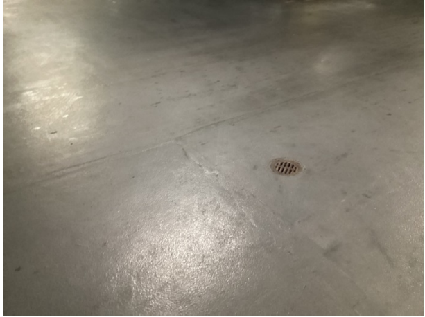
1P traffic coating
