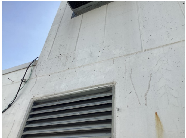
Repaired cracks at penthouse
