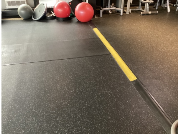
Flooring at exercise room
