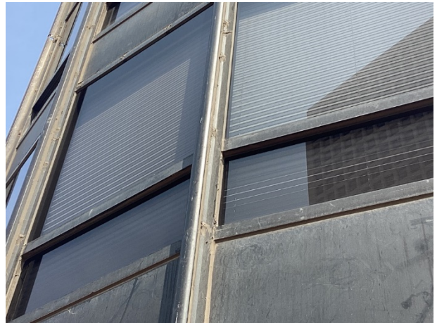
Sealants at metal to metal and metal to glass
