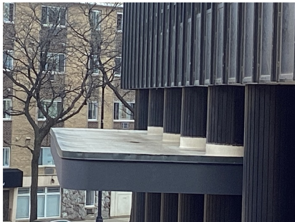
Lobby canopy roof
