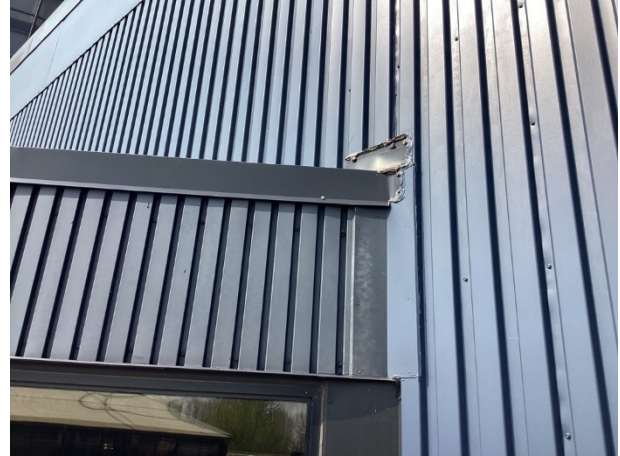
Metal siding at transition
