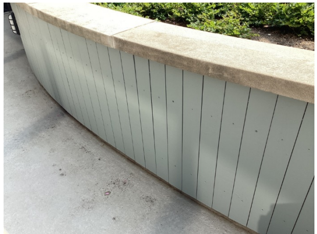
Siding at planter
