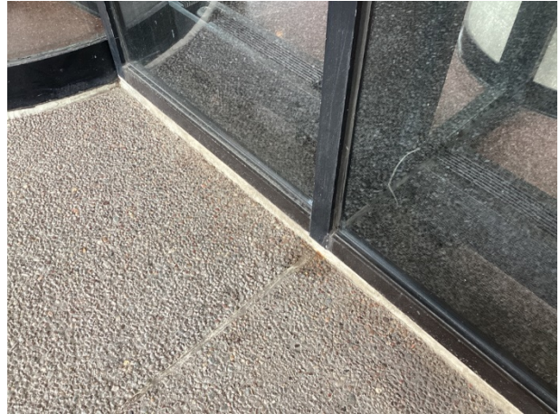
Lobby window system
