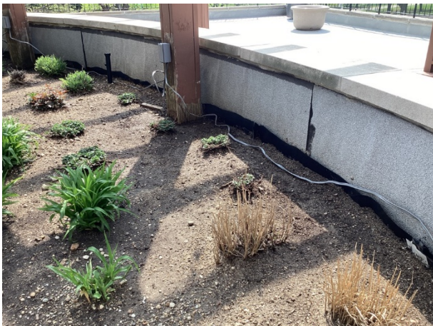
Perimeter at planter at 2nd floor
