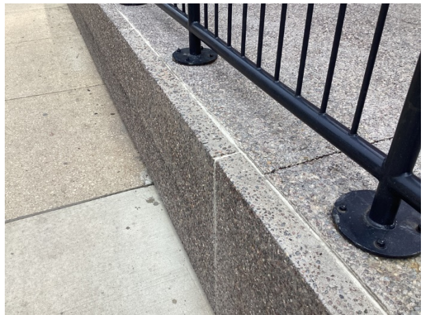
Perimeter at plaza
