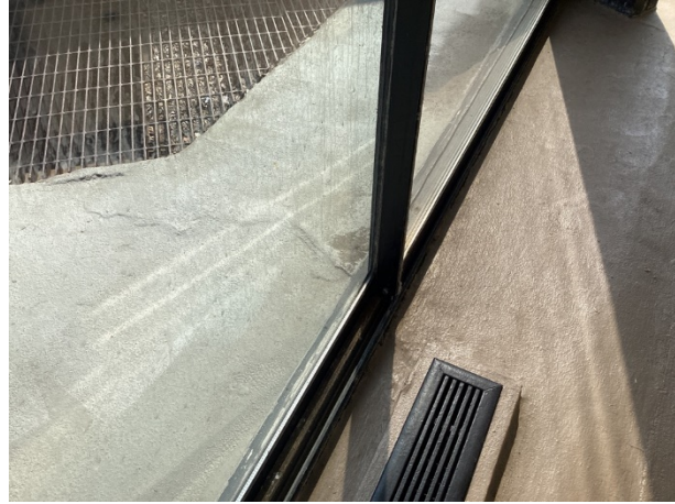
Pool area sliding door
