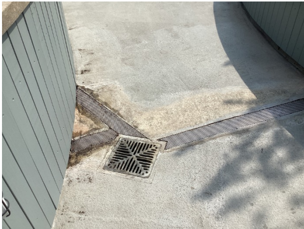
Modifications at drain at 2 nd floor concrete
