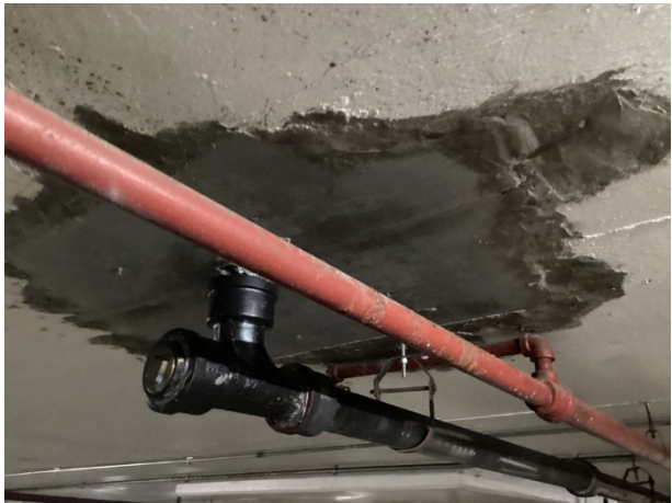
Concrete repairs beneath 1P
