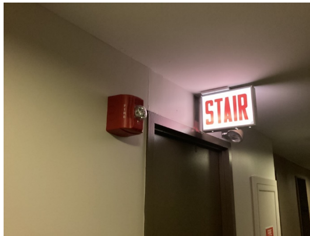
Fixtures at hallway
